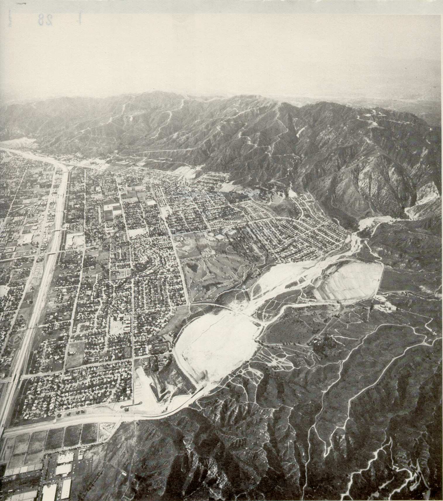
Lopez Dam and Reservoir (view from downstream of dam, taken 5/14/85).
