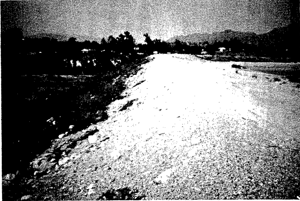
(a) Downstream Slope.
