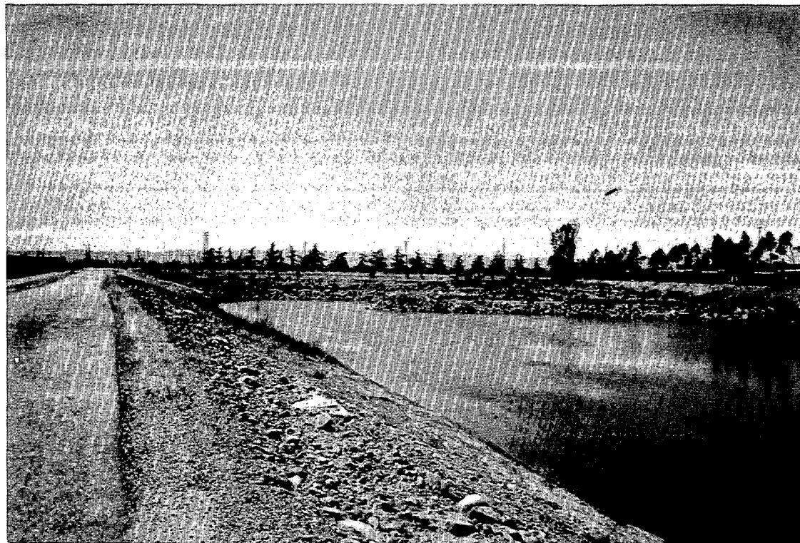
Figure 3-2. Hansen Spreading Grounds' Infiltration Pond.
