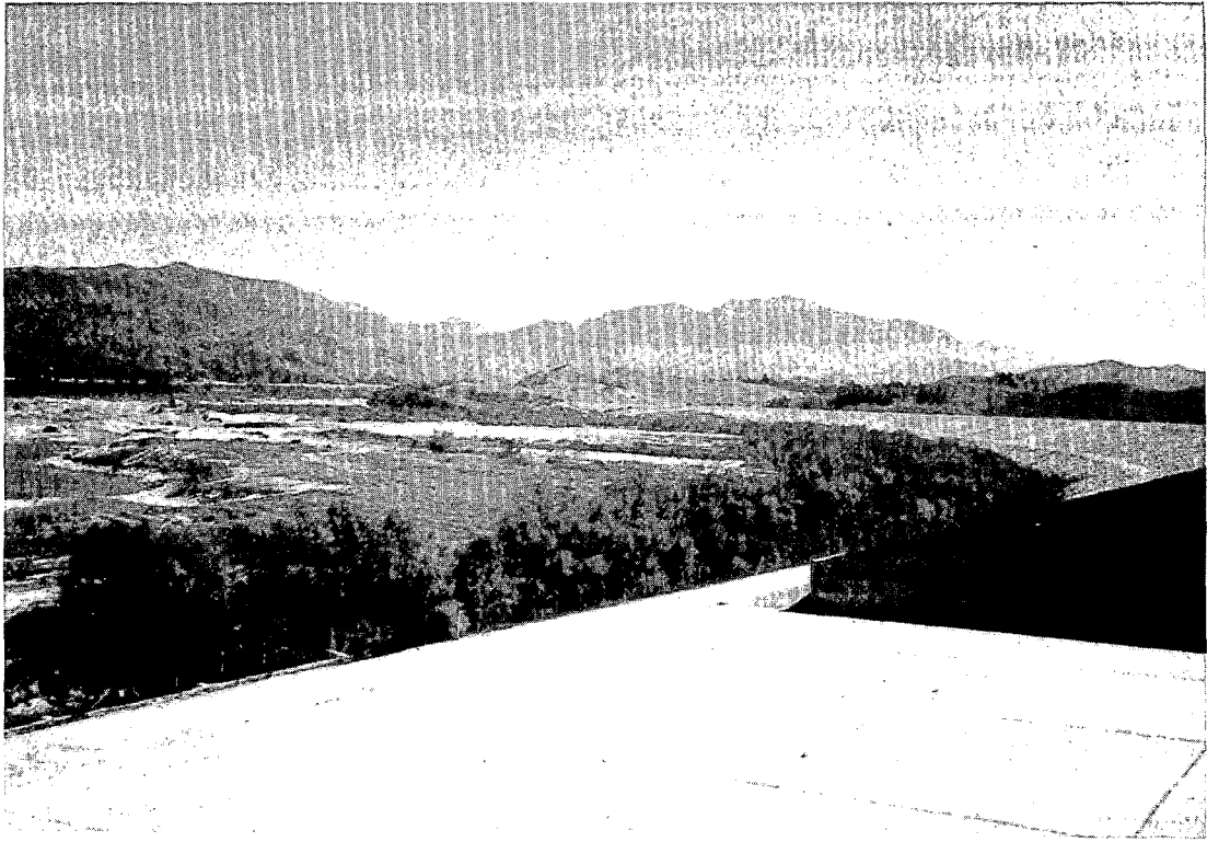
Figure 2-1a. Upstream View of Hansen Dam Embankment, Looking Northeast
