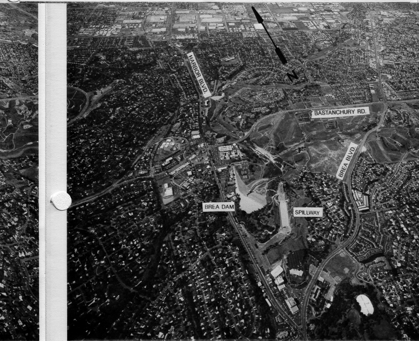
Photo of Brea Dam.
