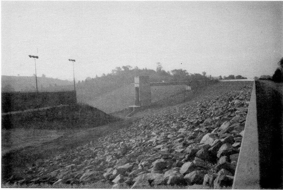
Photo No. 2-01. Upstream slope of dam (view toward southeast).
