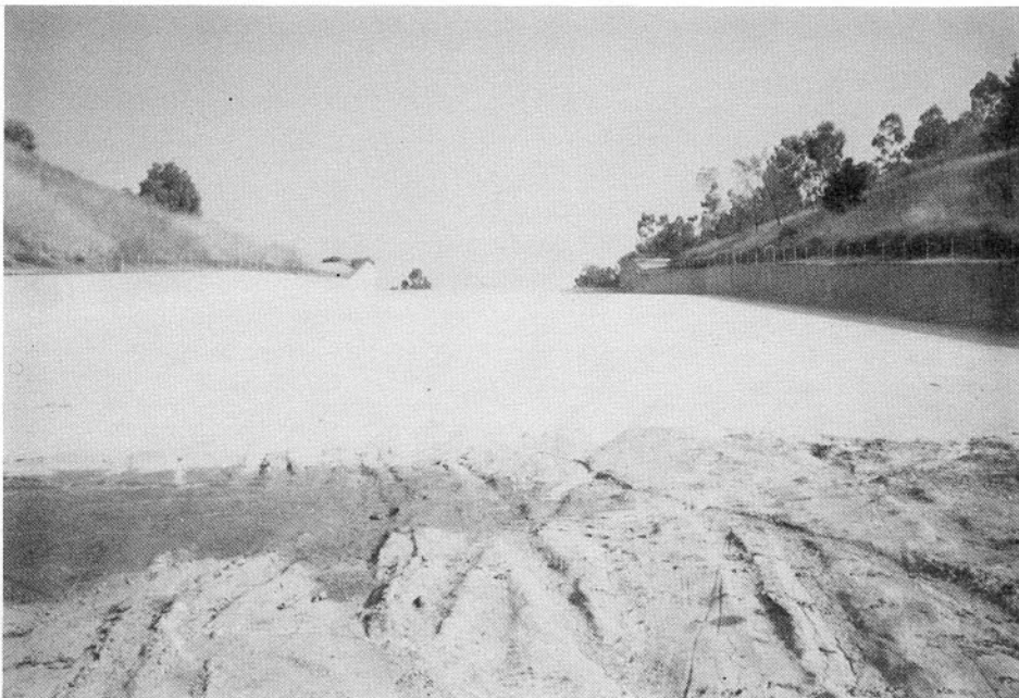
Photo No. 2-06. Spillway outlet channel (view looking upstream)
