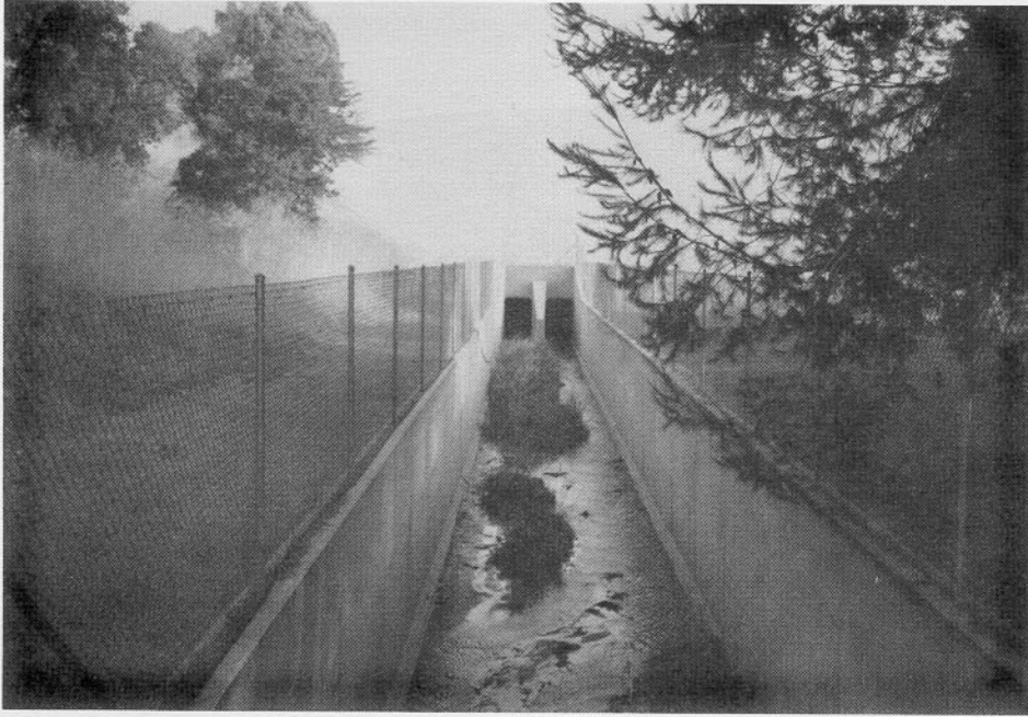
Photo No. 4-01. Brea Dam rectangular concrete outlet channel (view toward upstream).
