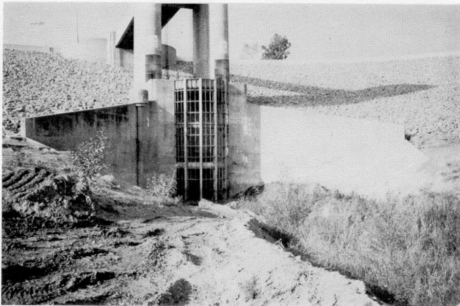
Photo No. 2-04. Outlet works: approach channel and trash rack (view toward downstream).
