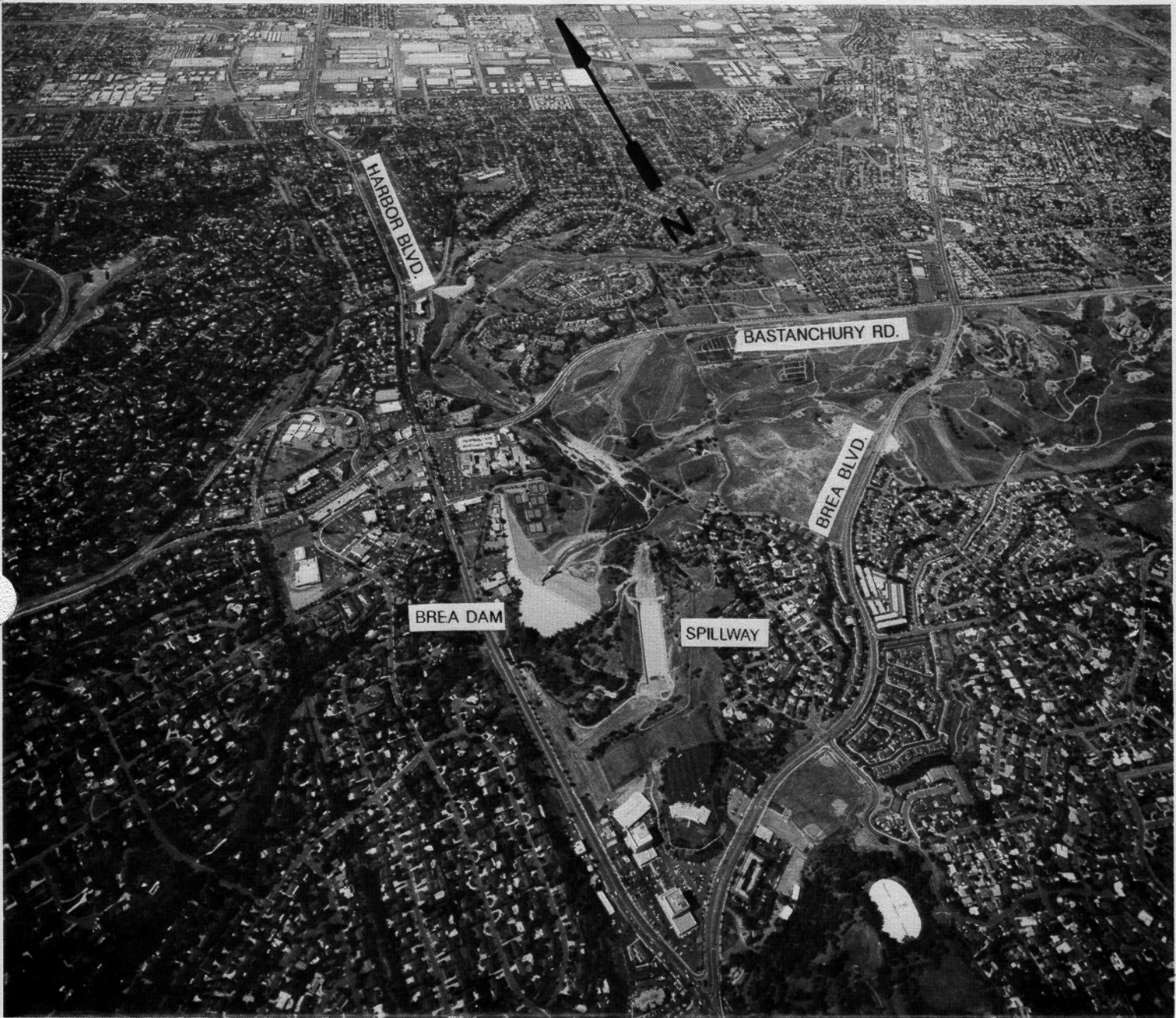
Photo of Brea Dam.
