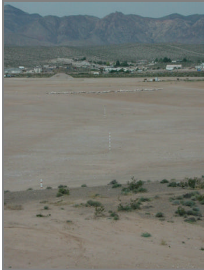
Photo 14. Blue Diamond Detention Basin . Sediment staff gages.
