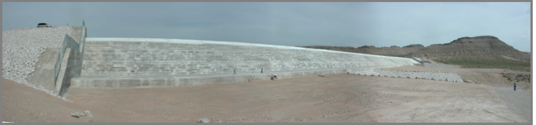
Photo 1. Blue Diamond Detention Basin . Spillway structure.
