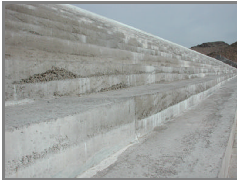
Photo 2. Blue Diamond Detention Basin . Spillway steps.
