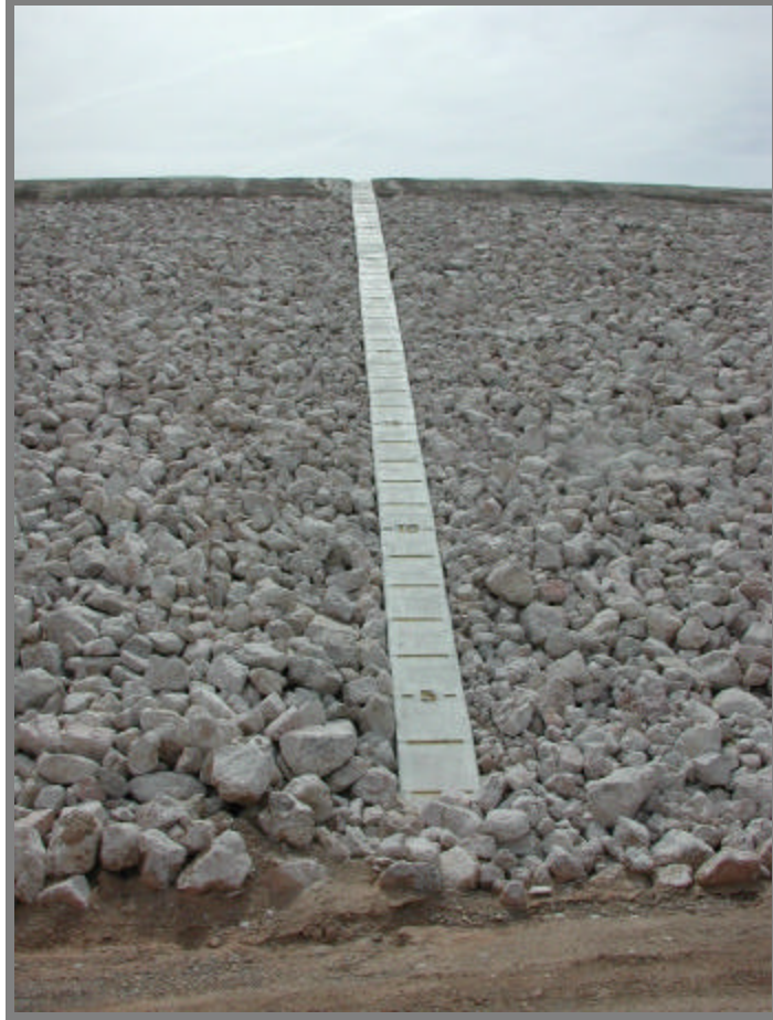
Photo 11. Blue Diamond Detention Basin . Basin depth gage.
