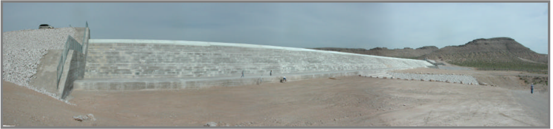
Photo 1. Blue Diamond Detention Basin . Spillway structure.
