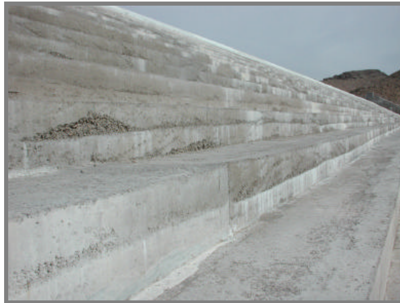
Photo 2. Blue Diamond Detention Basin . Spillway steps.
