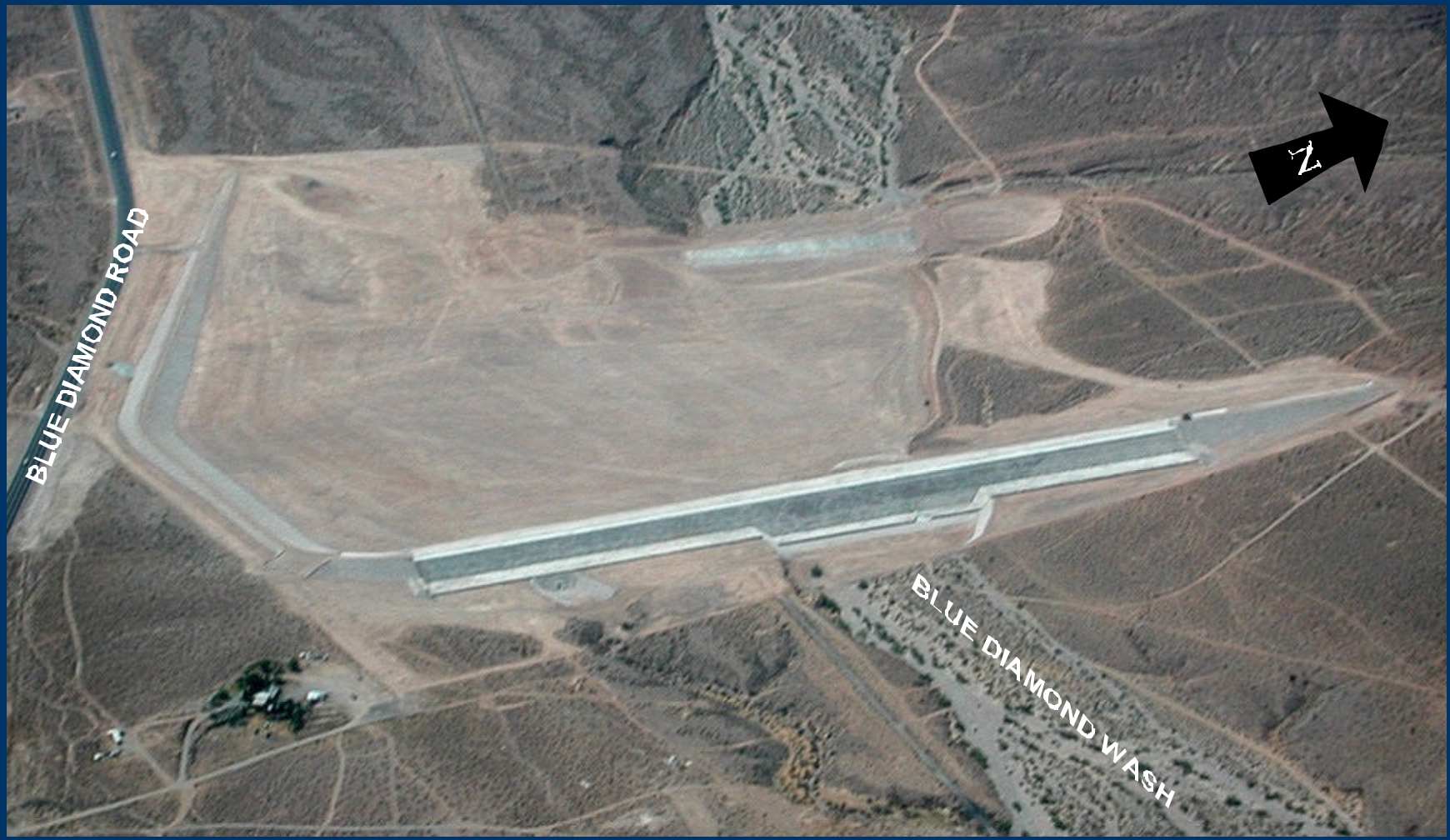
Blue Diamond Detention Basin – 15 May 2001
