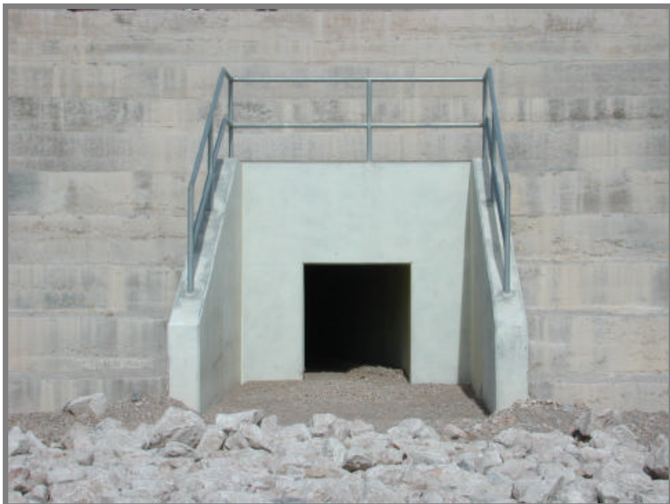
Photo 9. Blue Diamond Detention Basin . Downstream end of basin bypass conduit.
