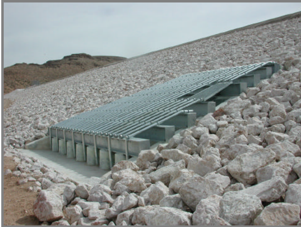
Photo 4. Blue Diamond Detention Basin . Outlet works trash rack.
