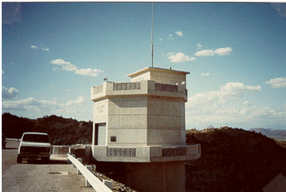
Photo 5-02. Alamo Dam control house.
