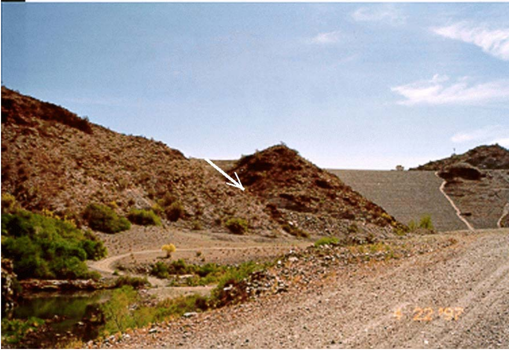
Photo 2-05. Gully (arrow) through which spillway flows discharge before rejoining Bill Williams River channel.
