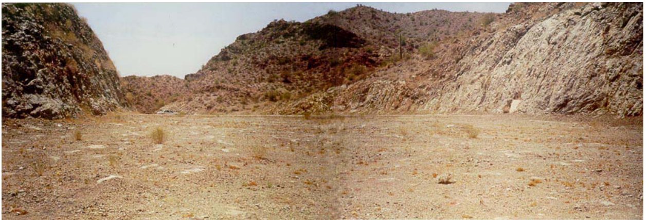
Photo 2-04. Spillway channel looking downstream.
