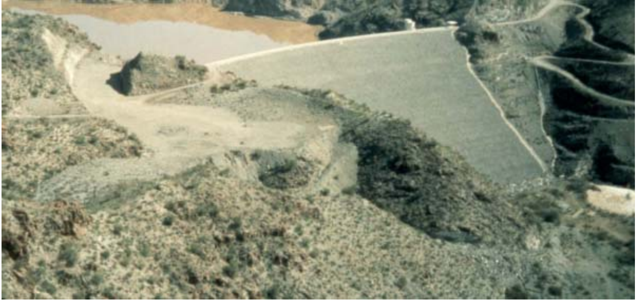
Photo 2-03. Aerial view of spillway adjacent to right abutment of dam.
