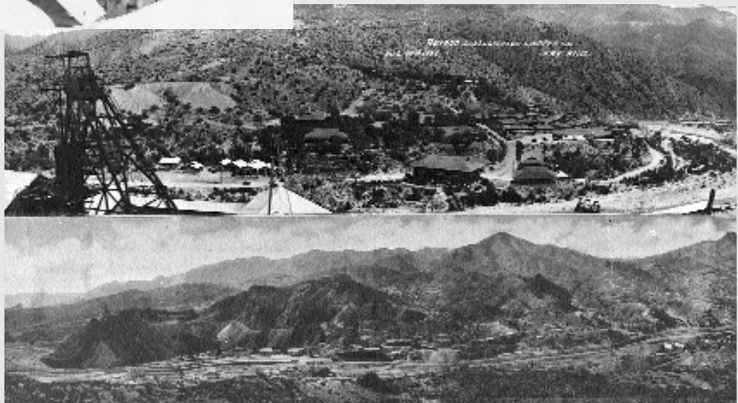
These two panoramic views of the mining town of Ray, Arizona show the more pleasant company houses at upper right and the neighborhood of "Sonora" in the lower view tucked in a notch in the mountain at center. Like many historic mining locations related to Hispanics, all evidence of "Sonora" has disappeared under the Ray open pit mine.
