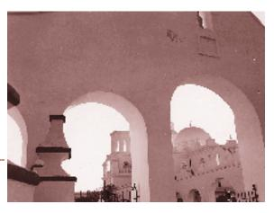
shaped them, fired them, and laid them in lime mortar to form the walls and multi-domed ceiling. They excavated, burned, and slaked the lime. They hauled rocks to the site for use in foundations and in the cores of walls. And when the job was finished in 1797, they worshiped in the building even as their descendants do to the present.
