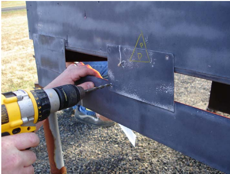
Figure B-4. Removing Rivets From Older Outer Baffles
