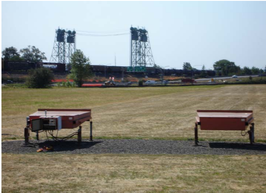
Figure B-1. Interstate I-5 Bridge Forming Obstruction
