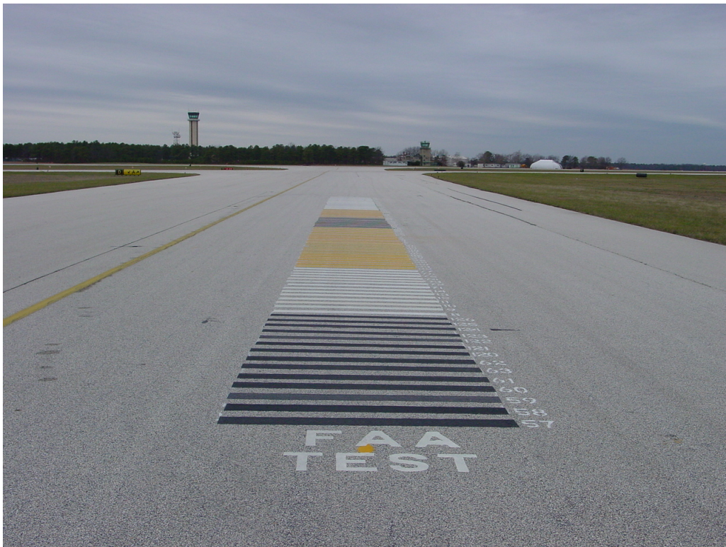
FIGURE 7. LINES AT TAXIWAY DELTA ON OLD HOT-MIX ASPHALT
