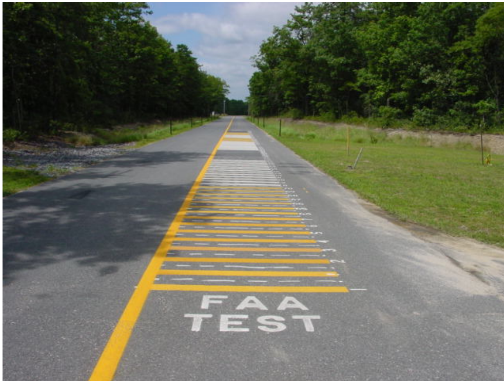
FIGURE 5. LINES AT NEWER HOT-MIX ASPHALT TEST SITE (Pavement Placed 1999)
