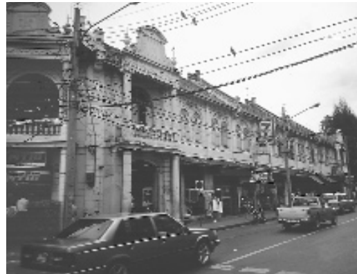
Historic shophouses in Bangkok, Thailand. Subject for the 1997 and 1998 University of Hawai'i Asian Preservation Field Schools. Photo by William Chapman.
