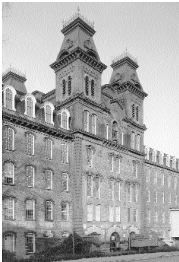
Harmony Manufacturing Co. Mill No.3, central block, west face; quoins are cast iron. Photo by Jack E. Boucher.
