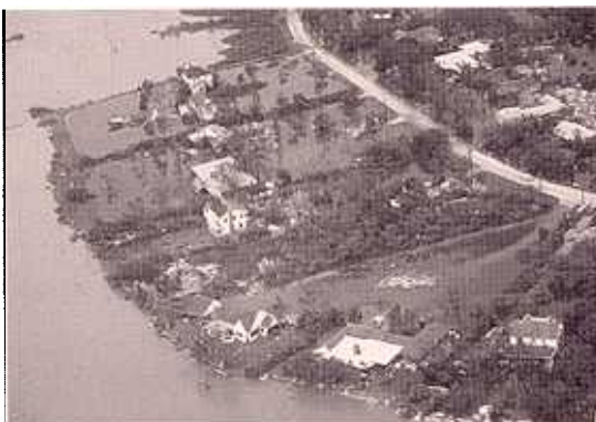
Subsidence allowed Alicia's storm waters to wash in and flood these homes in the Baytown area.
