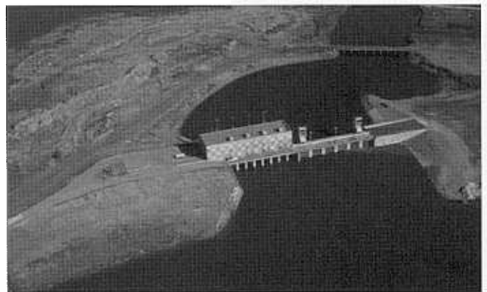
The pump station on Port Arthur Hurricane-Flood Protection System moves floodwaters out of Alligator Bayou.
