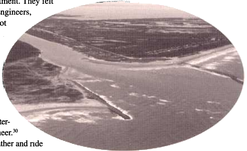
Jetties guard the mouth of the Colorado River from shoaling.
