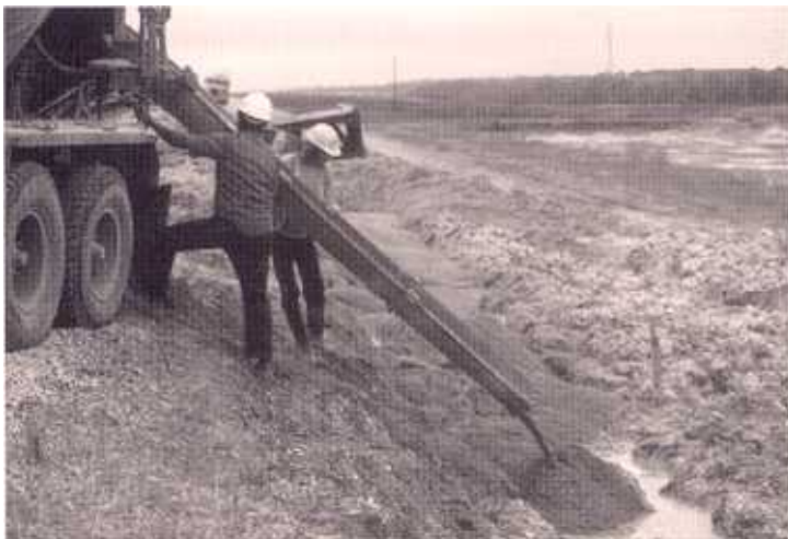
Reinforcing drilling “mud” flows into Addicks Dam slurry trench.
