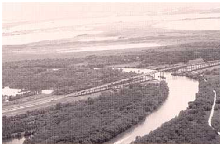
In May 1987, the court gave the go-ahead to proceed on Wallisville after 15 years of delay. Interstate 10 and the reservoir can be seen in the September 1987 photo.
