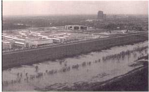
Right: Water collects behind Addicks Dam after heavy rains.
