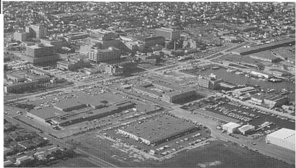
Right: The Essayons Building was located between the ship channel and The University of Texas Medical Branch on the east end of Galveston Island.
