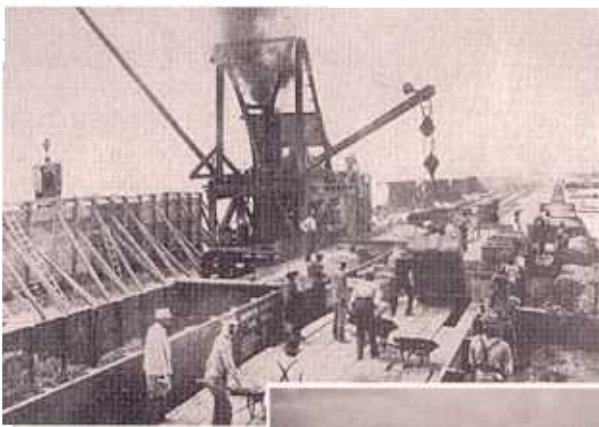
Above: An early photo shows seawall construction.
