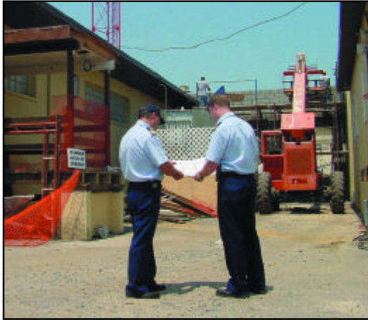
LTJG Ken Shovlin, Facilities Design and Construction Center Pacific, Seattle, Washington, and LCDR Engblom, Loran Support Unit, Wildwood, New Jersey, examine the construction of a new transmitter lab facility at the Loran Support Unit. The facility will house the next generation of Loran transmitting and timing equipment currently in development. The base of the 625 foot tall
