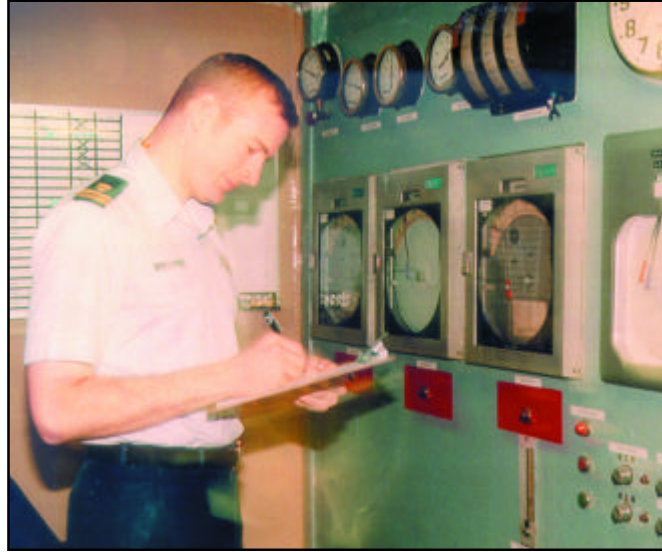
LTJG Alex Dodd, a 1998 graduate of the Coast Guard Academy, monitors power output gauges in the boiler plant at the Coast Guard YARD in Baltimore, Maryland. LTJG Dodd holds a Bachelor of Science degree in Civil Engineering.
