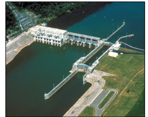
Cordell Hull Lock and Dam, a run-of-river project (TN)
