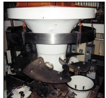
New turbine being installed at Bonneville Dam (OR)
