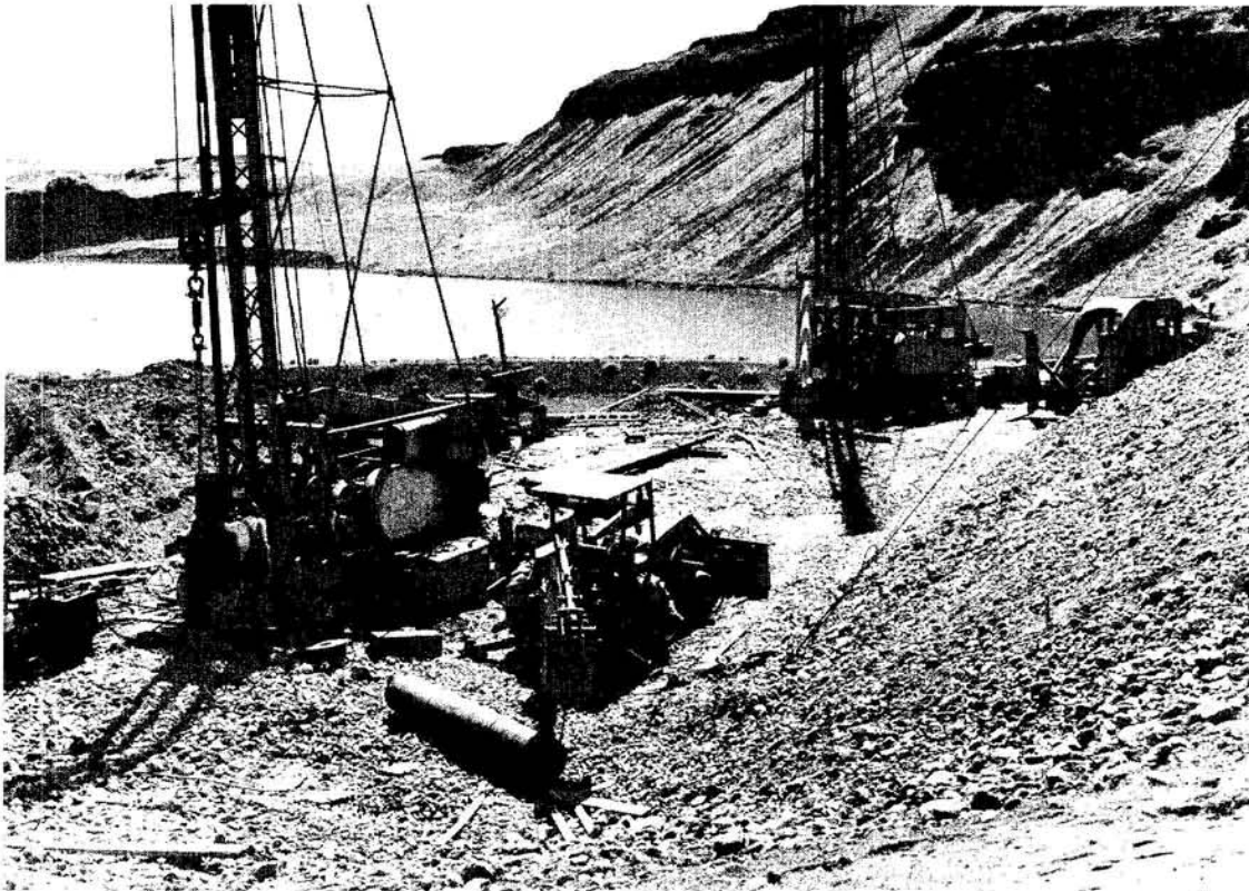
FISH HATCHERY TEST WELL DRILLING AT THE LYONS FERRY SITE
