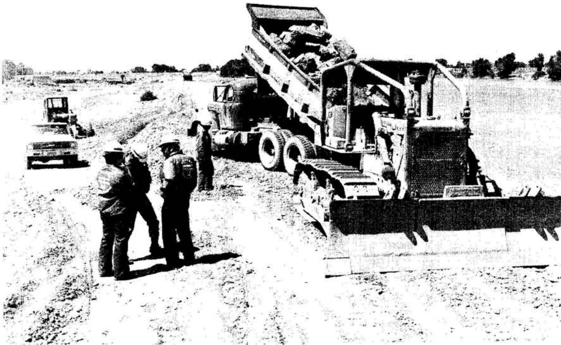
HANK VAN SCOTTER AND LIEUTENANT LANE GRIFFEN SUPERVISE LEVEE BUILDING
