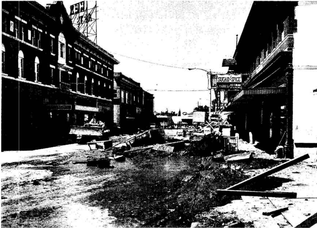
DEBRIS CLEANUP AT REXBURG
