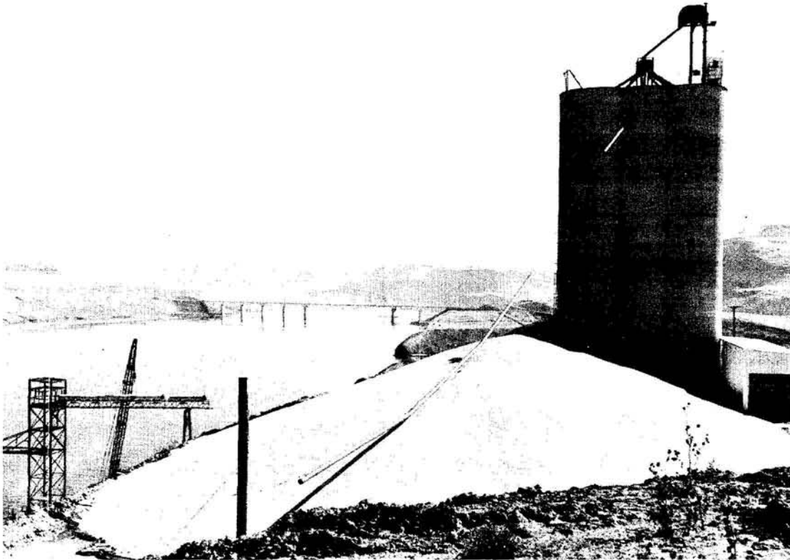
PORT OF COLUMBIA GRAIN ELEVATOR
