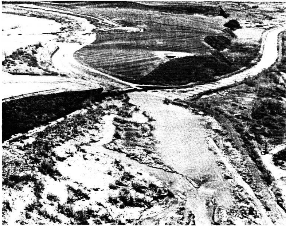
MILL CREEK PROJECT IN ACTION Offstream Reservoir at Extreme Left
