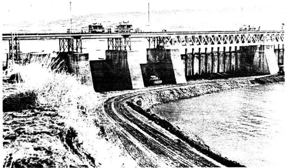
REMOVAL WASHINGTON WATER POWER DAM
