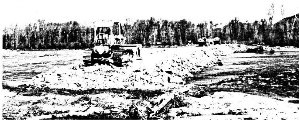
FLOOD FIGHT ACTION - JACKSON, WYOMING - 1975 Cut-off Dike to Preclude Avulsion
