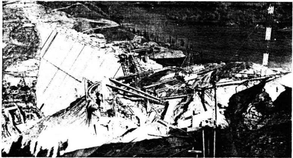
DWORSHAK DAM CONSTRUCTION - NOVEMBER 1971 POOL BEING RAISED - POWERHOUSE UNDER CONSTRUCTION
