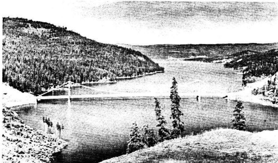
DENT BRIDGE (River Mile - 17)
