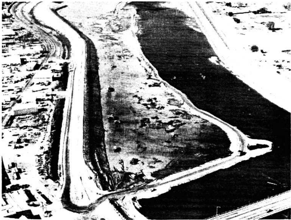
CLEARWATER RIVER - MEMORIAL (16TH STREET) Bridge Downstream - Levee and By-Pass Road Along Lewiston Waterfront Holbrook Island Excavation Center of Picture North Bank Levee in Place
