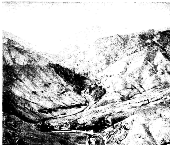
TWIN SPRINGS DAMSITE - BOISE RIVER (QUARRY AREA - LEFT SIDE OF PICTURE)
