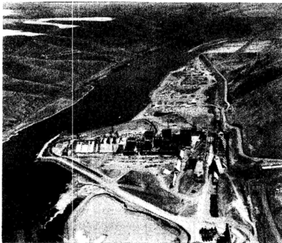
1st-STEP COFFERDAM - OCT 1968
