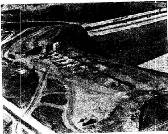
SPILLWAY CREST UNDER CONSTRUCTION
