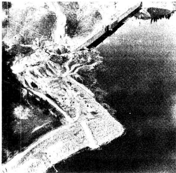
LOG HANDLING AREA AT LEFT ABUTMENT POOL PARTIALLY RAISED WITH CONSTRUCTION STILL IN PROGRESS
