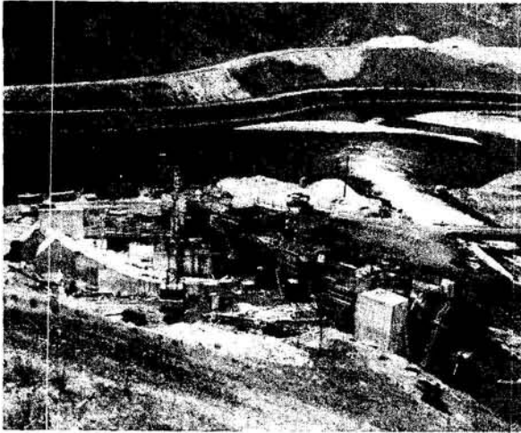
OUTLET WORKS WITH FLIP BUCKETS ON LEFT
