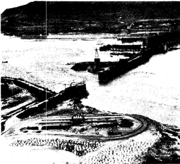
OREGON SHORE COFFERDAM READY TO CLOSE GAP IN CELLS NOTE TETRAHEDRONS IN FOREGROUND
