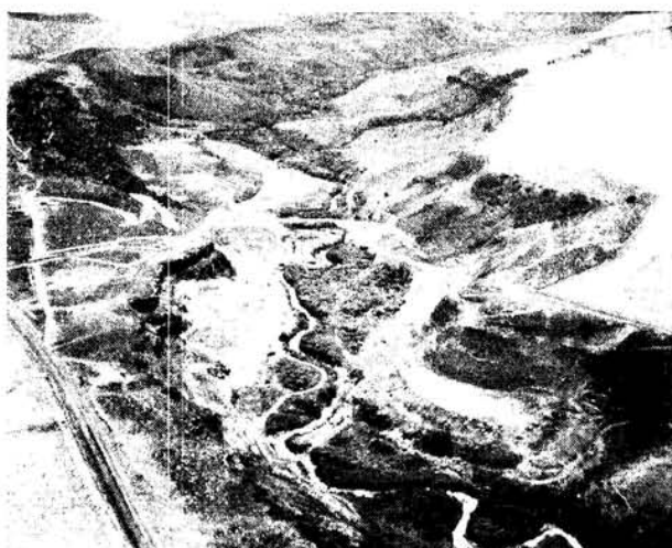
RIRIE DAMSITE - SEPTEMBER 1967
