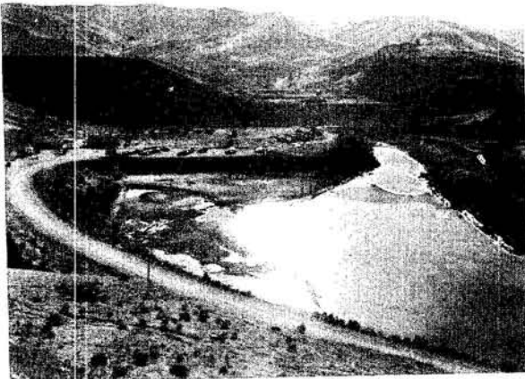
DIVERSION CHANNEL CLOSED; DAM CONSTRUCTION UNDERWAY
