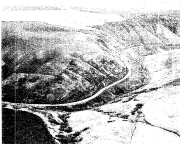
ACCESS ROAD - POMEROY TO DAM DECEMBER 1966
