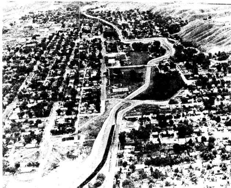
PORTNEUF RIVER THROUGH POCATELLO - BEFORE AND AFTER CHANNELIZATION - LOOKING UPSTREAM
