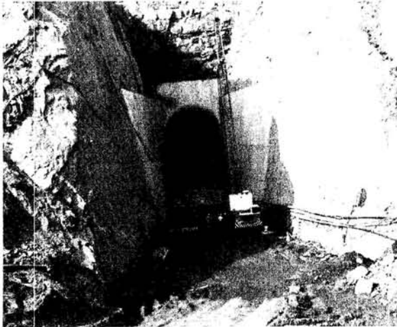
UPSTREAM DIVERSION TUNNEL PORTAL
