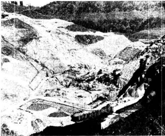
DAM BASE WITH DRAFT TUBES - OCT '68
