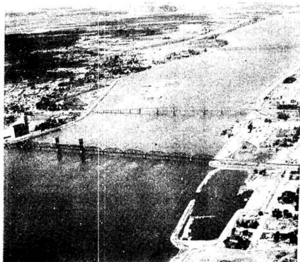
PASCO - KENNEWICK LEVEES HARBOR FRONT AND BRIDGES (NPRR IN FOREGROUND)
