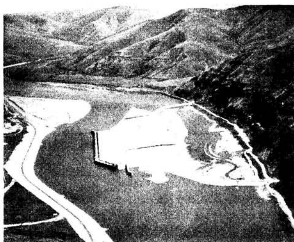
LOWER GRANITE DAM - 1967
