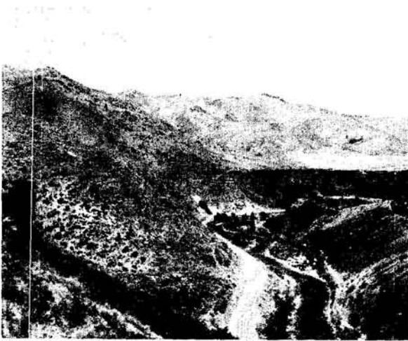
MORES CREEK CANYON BEFORE BRIDGE CONSTRUCTION
