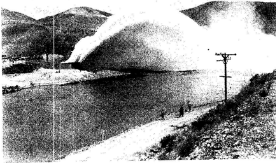
OUTLET WORKS IN OPERATION
