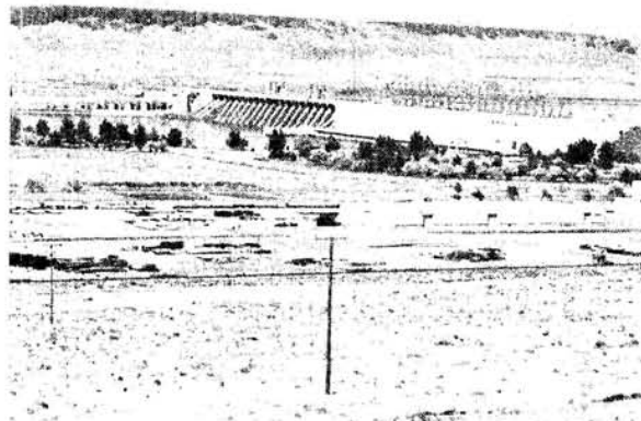
THE COMPLETED PROJECT
