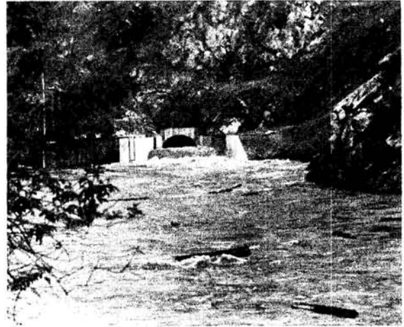
TUNNEL EXIT WITH FISH CHANNEL AND TRAP ON LEFT
