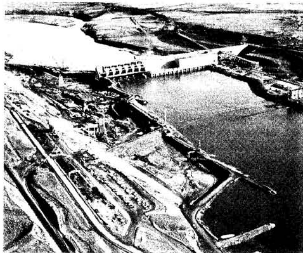
SECOND STEP - NORTH SHORE COFFERDAM WORK - 1960
