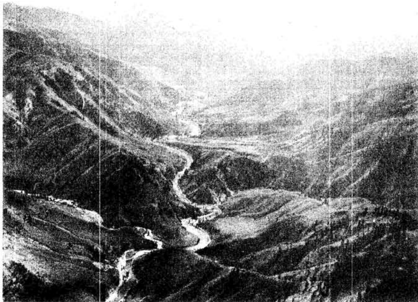
TWIN SPRINGS DAMSITE UPSTREAM OF ARROWROCK RESERVOIR (DAMSITE IN CANYON SECTION, CENTER OF PICTURE)
