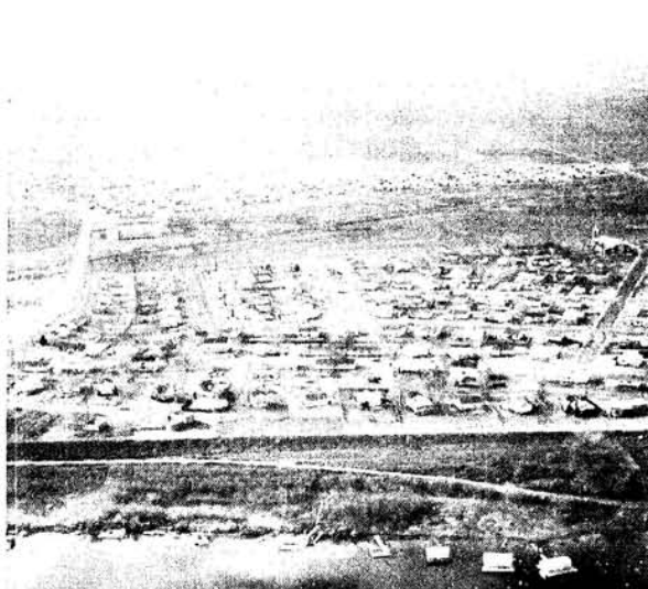
RICHLAND LEVEE AND WATERFRONT
