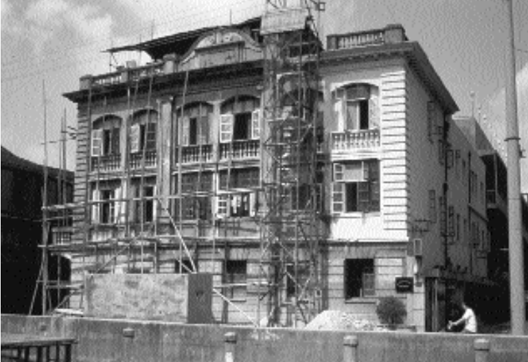
Warehouse being repainted, Shanghai.
