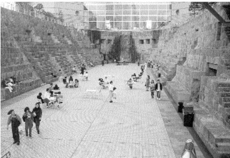
Former dry dock, Yokohama, Japan, 1994. People now can stroll in a public plaza where once ships for the Japanese Navy were built. Photo by the author.
