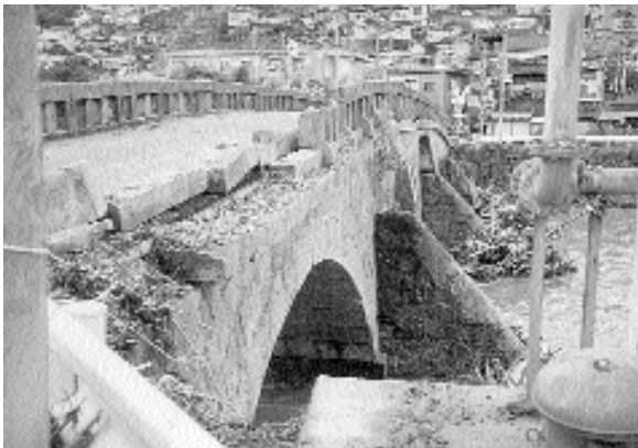
Tamae bridge, 1849, under demolition, Kagoshima, Japan, 1994. Photo by Takashi Itoh.
