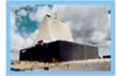
Early Warning Radar
