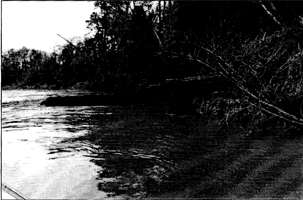
FIGURE 2: View downriver of one chine log extending out of the river bank and over the Neches River.
