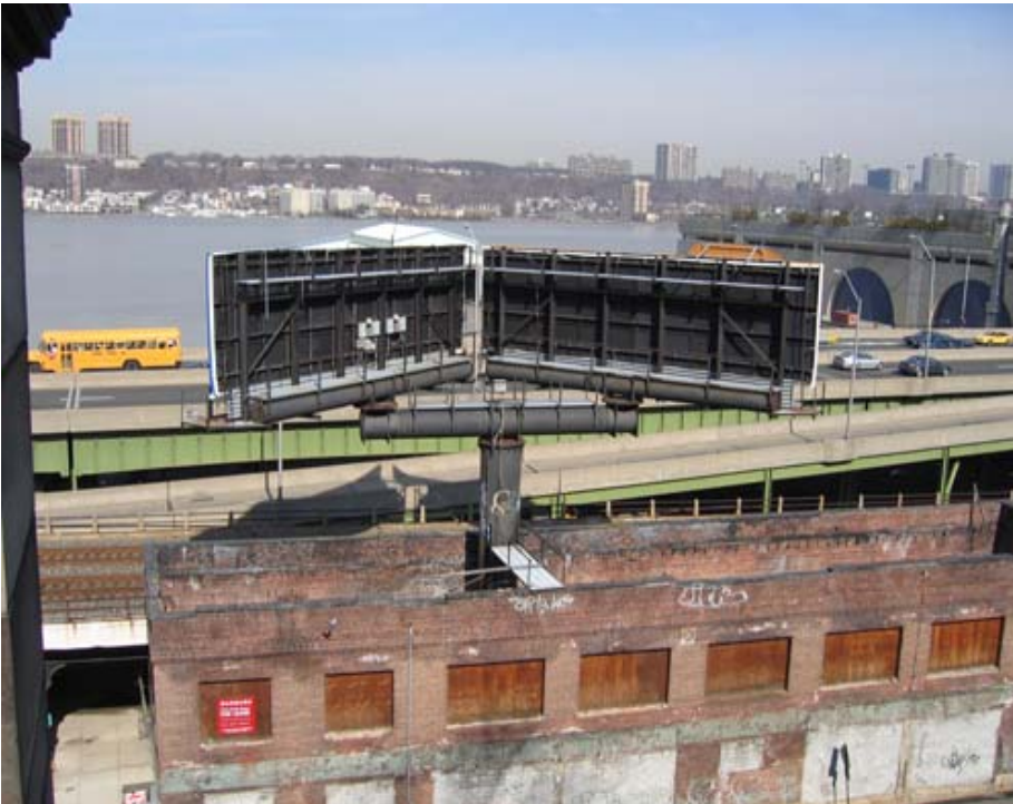
Scenic and sweeping views have given way to blighted buildings and obtrusive billboards and signage
