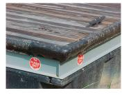
boaters of docks lining the shore. A boat versus dock collision can be expensive and deadly. Second, the reflectors are important to boaters so they can find the correct location of the dock at night. Docks with an unusual array of more than four reflectors serve as good landmarks to the boater navigating at night.
