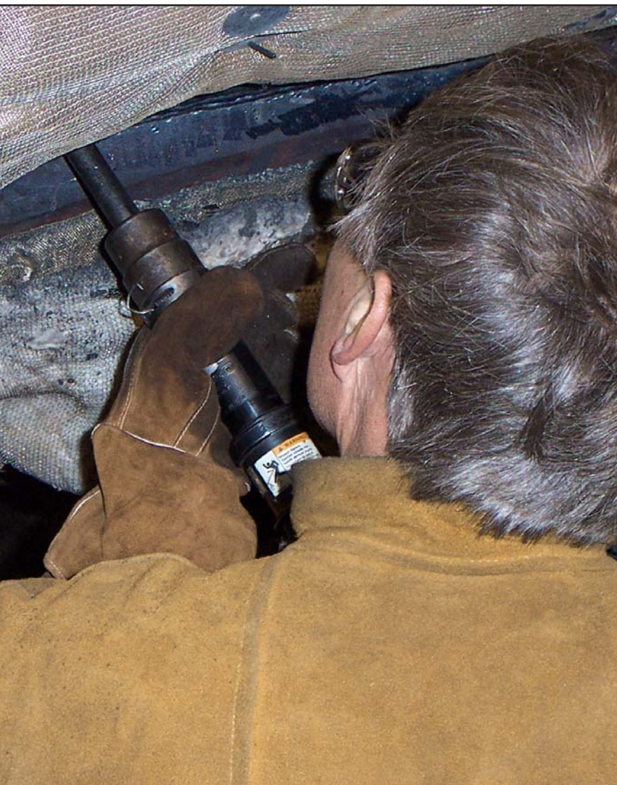
Above, Pat Marsh, crane operator, uses a forklift to take the recovered blade section to a nearby welding area (photo by Jim Hay). Left, Carey Basel, welder, grinds and welds on the blade section, shaping the broken edge for reattachment to the turbine (photo by Sam Liming).
