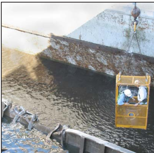
Ice Harbor workers move the bulkhead into position so the Empress of the North can leave the navigation lock.
