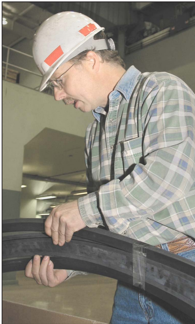
Above-left, Power plant mechanics at Lower Monumental Lock and Dam, use screwdrivers to pry out the old, fibrous-material oil seal from the Unit 4 turbine (photo by Sue Walton). Above-right, Ron Standing, power plant mechanic crew foreman at the dam, examines one of the new rubber seals that his crew will install on the Unit 4 turbine (photo by Gina Baltrusch).
