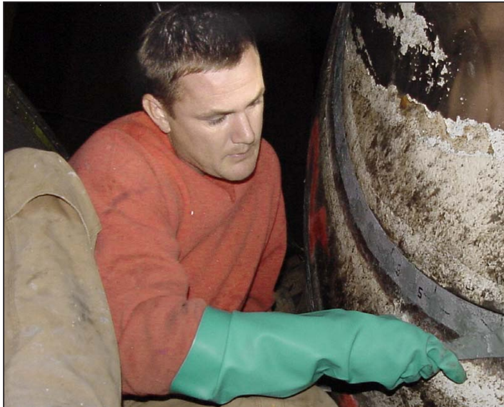
Jamie Munson, a painter, caps off the bolt holes of the followers with putty and epoxy to p
