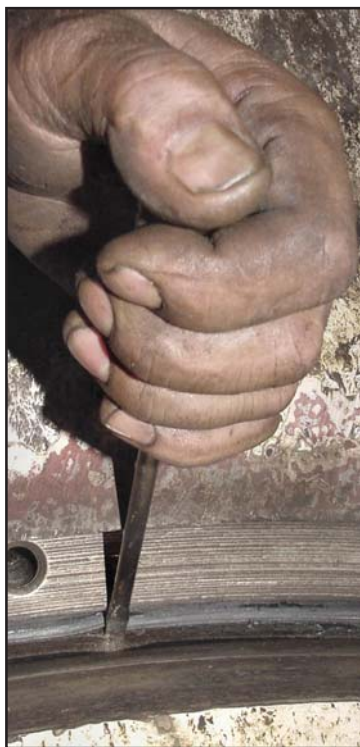
Above-left, Power plant mechanics at Lower Monumental Lock and Dam, use screwdrivers to pry out the old, fibrous-material oil seal from the Unit 4 turbine (photo by Sue Walton). Above-right, Ron Standing, power plant mechanic crew foreman at the dam, examines one of the new rubber seals that his crew will install on the Unit 4 turbine (photo by Gina Baltrusch).
