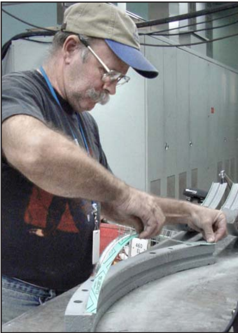
After cleaning the followers to remove the past year's build-up of rust and grime, Richard Spooner, power plant mechanic, applies a thin, rubber-like material that will create a washer-like sealing effect once the followers are reinstalled over the new oil seals (photo by Sue Walton).
