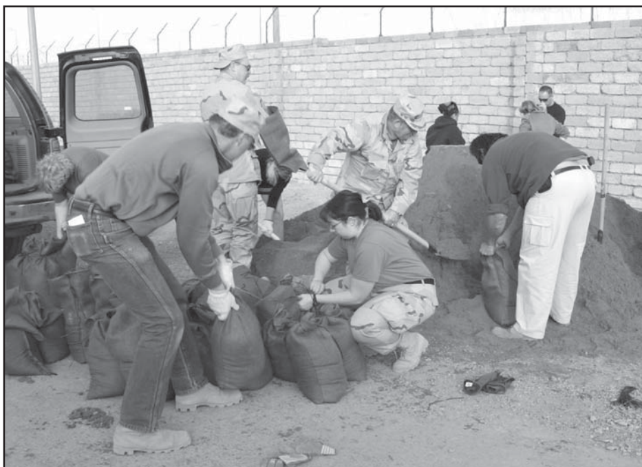
Photos by Nola Conway, Gulf Region North District
