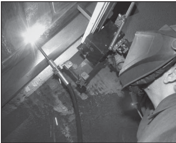
The track-mounted, automated welder applies smooth, even lines of new stainless steel.
