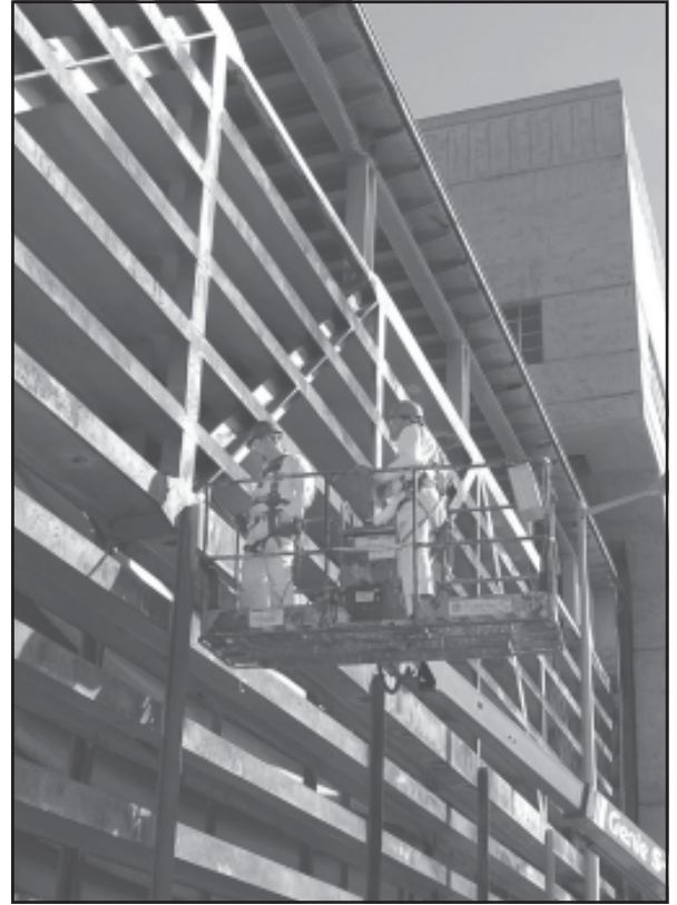
Welders from Inland Industrial Rigging repair cracks and broken welds in the downstream navigation lock gate at Lower Monumental Lock and Dam.
