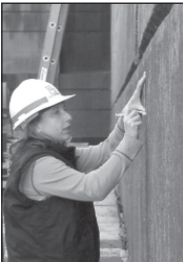
Above, Margie McGill, project manager, marks the walls inside Lower Monumental Dam's navigation lock for drilling core samples. Right, Little Goose Dam workers, Tony Sijohn, (left) powerhouse mechanic, and Tim Collier, (right) rigger, guide a diver into the downstream navigation lock channel to inspect for debris.
