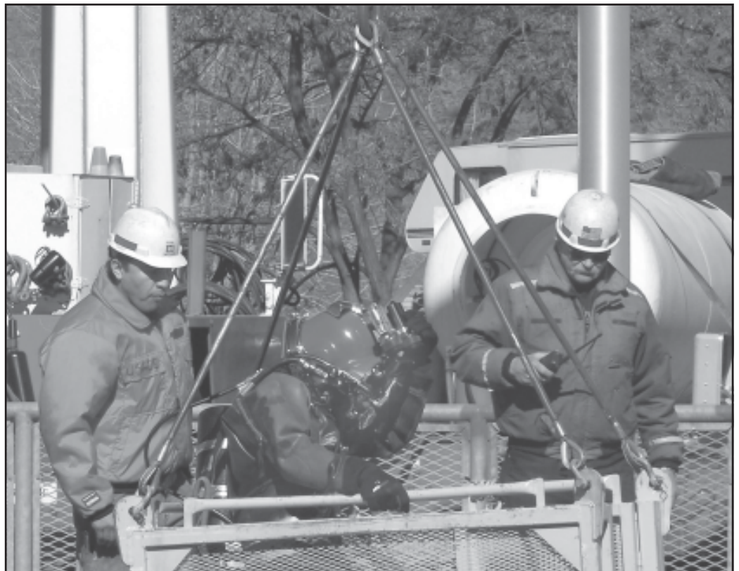
Welders from Inland Industrial Rigging repair cracks and broken welds in the downstream navigation lock gate at Lower Monumental Lock and Dam.
