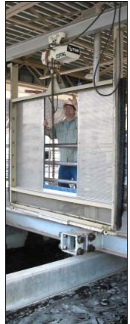
Ches Brooks, a biological science technician at Lower Monumental Dam, uses a gantry crowder to herd fish ready for barge transport out of the holding raceways.
