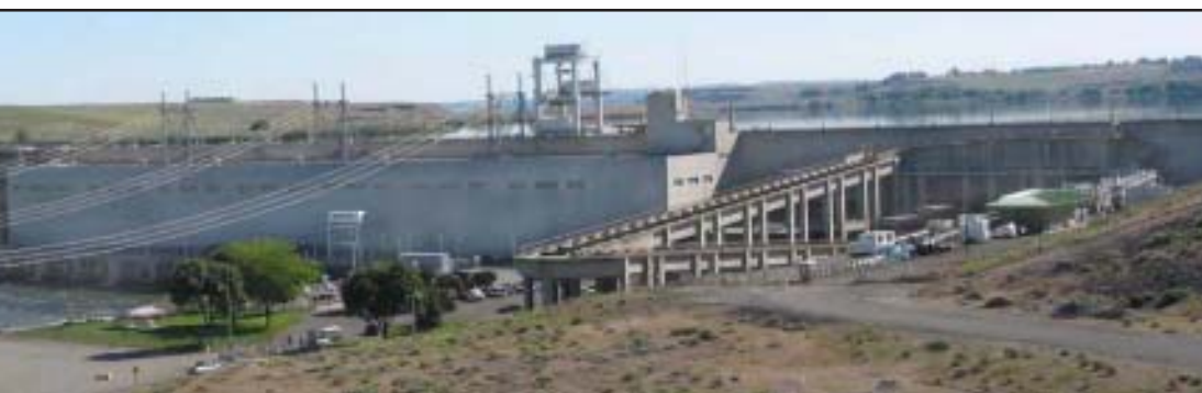
(The roofed building on the right) and back into the lower Snake River on the dam's downstream side.
