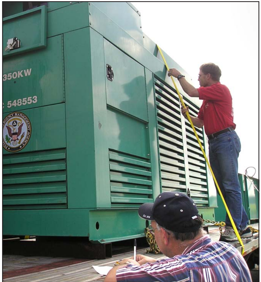
photo by Mike Deccio, engineering technician, Operations Division
