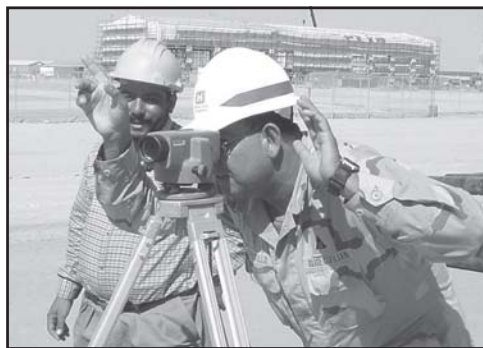
photo provided by Bert Cerrillo, Afghanistan Engineer District
