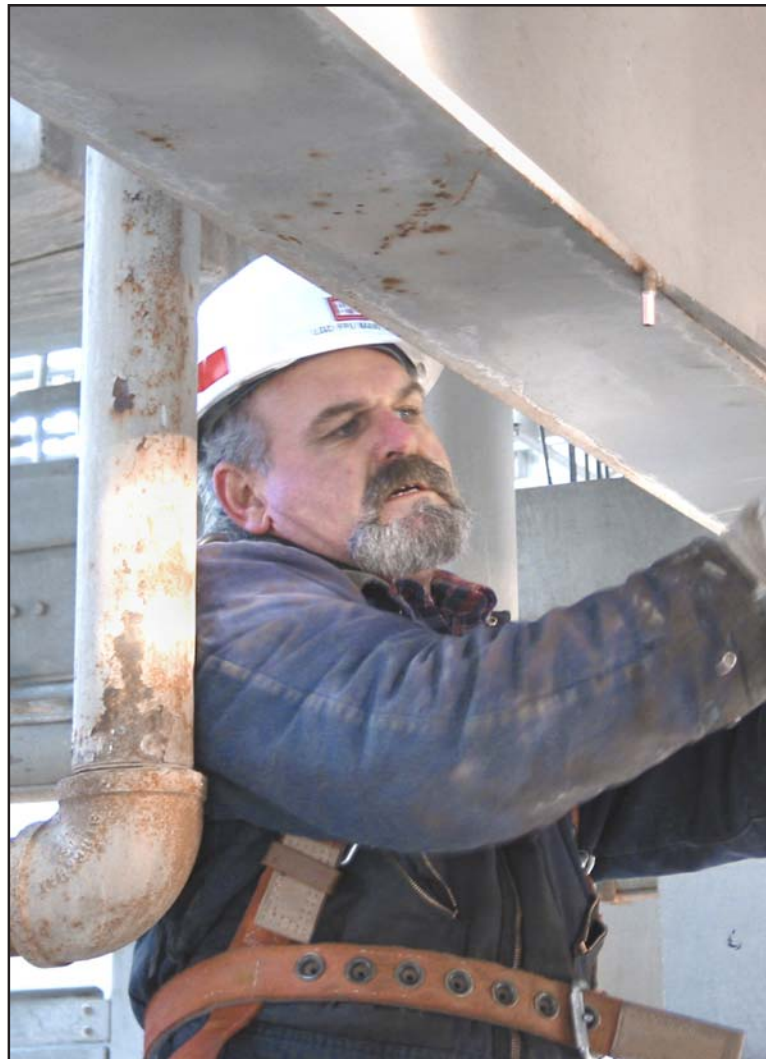
Roger Bowen, maintenance worker, repairs air lines that run to valves.
