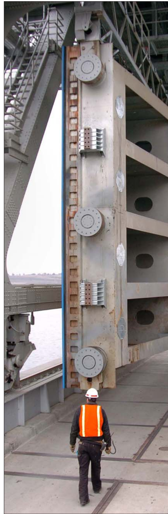
Above, Peter Stewart, a rigger at McNary Dam, moves a gate as it is moved by a gantry crane across the dam into a spillway slot. Left, Stewart (at left) and Terry Zerb, a representative from Walla Walla District's Construction Department, discuss the project which spillway to insert a newly refurbished gate.
