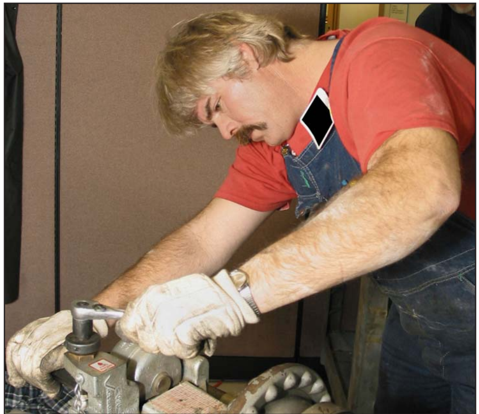
Dave Ogren, service technician foreman for Cascade Fire Protection, cuts new sections of pipe to repair the broken sections of the District headquarters building's fire-control sprinkler system.
