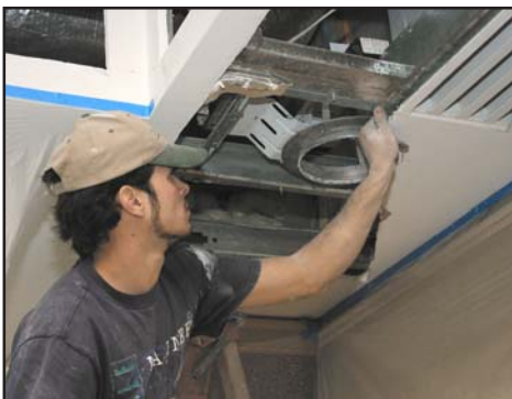
Dave Ogren, service technician foreman for Cascade Fire Protection, cuts new sections of pipe to repair the broken sections of the District headquarters building's fire-control sprinkler system.
