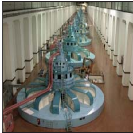
McNary's powerhouse today.
