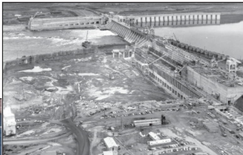
Above, McNary's navigation lock is complete (in the background), and the powerhouse and stilling basin are under construction in this 1953 photograph. Left, McNary Project today. Below, generator unit number 4 goes online.
