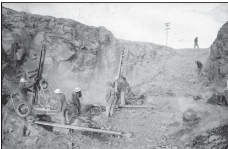
In 1948, work crews drilled into the riverbed to begin building the navigation lock.
