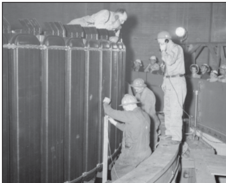
Powerhouse workers gather (far-right) to watch the final positioning of the generator rotor number 4 on April 23, 1954.
