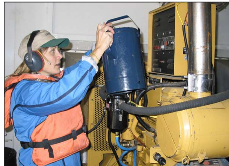
Above, Suzette Frazier, biological technician and 'barge rider,' adds oil to one of four engines that run pumps to keep water flowing in the holding tanks on the barge transporting smolts downstream. Barge riders tend the fish around the clock during the two-day trip downstream. Right, the tug boat, Mary Jane II, steers a barge full of young salmon and steelhead away from the fish facility dock at Lower Granite Lock and Dam on the lower Snake River. The fish take a nearly 300-mile trip downstream and are released just past Bonneville Lock and Dam on the Columbia River.
