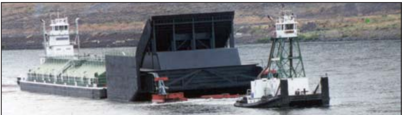
The Removable Spillway Weir was constructed at Vancouver, Wash., moved up the Columbia-Snake River system, and was installed at Lower Granite Dam in 2001. (PAO file photo)
