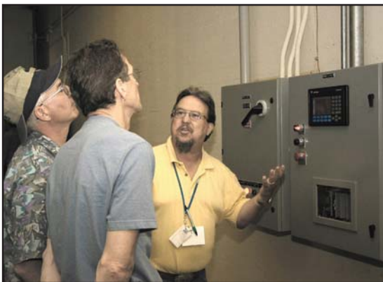
Herb Scheuerlein, a power plant electrician at McNary, explains how the turbine fish screens work. Right, workshop attendees representing numerous hydroelectric industry organizations from throughout the Northwest, watch Don Krueger, from General Electric in Portland, Ore., demonstrate a new welding technique on a scale model of turbine wicket gates.
