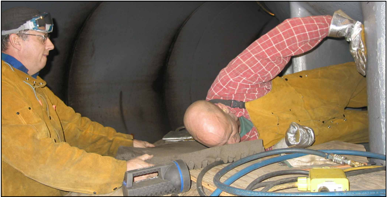
Sonny Mitchell, a utility worker at Dworshak, helps Bill Alteneder, a maintenance worker from Lower Granite, squeeze out from between the wicket gates of a Francis turbine at Dworshak's powerhouse.
