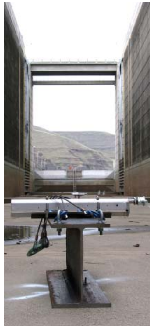
U.S. Geological Survey researchers installed course bubble diffusers mounted on I-beams in the bottom of the navigation lock at Lower Granite Lock and Dam to conduct in-water testing for the Chicago Underflow Plan. (Photo by Gina Schwetz)
