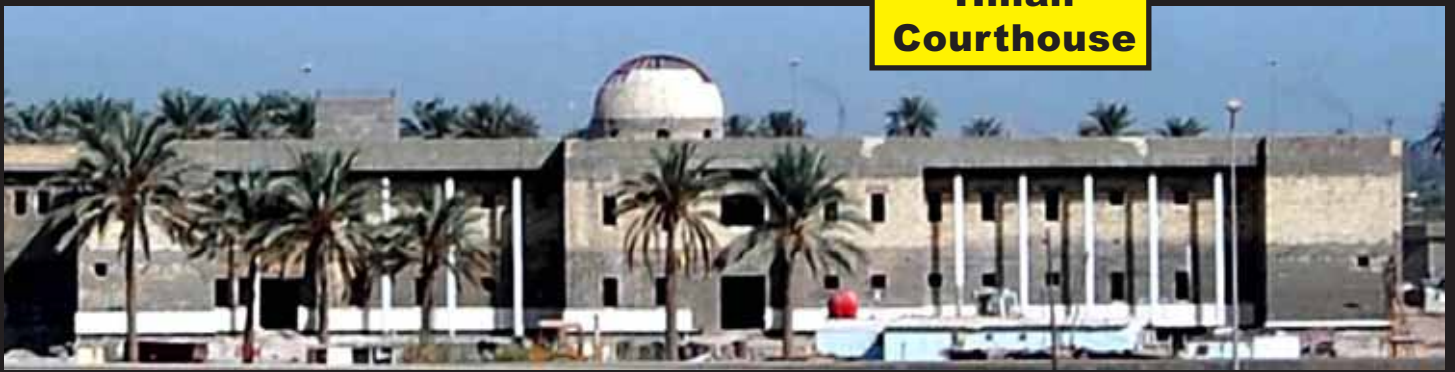
New Hillah Regional Courthouse under construction.
