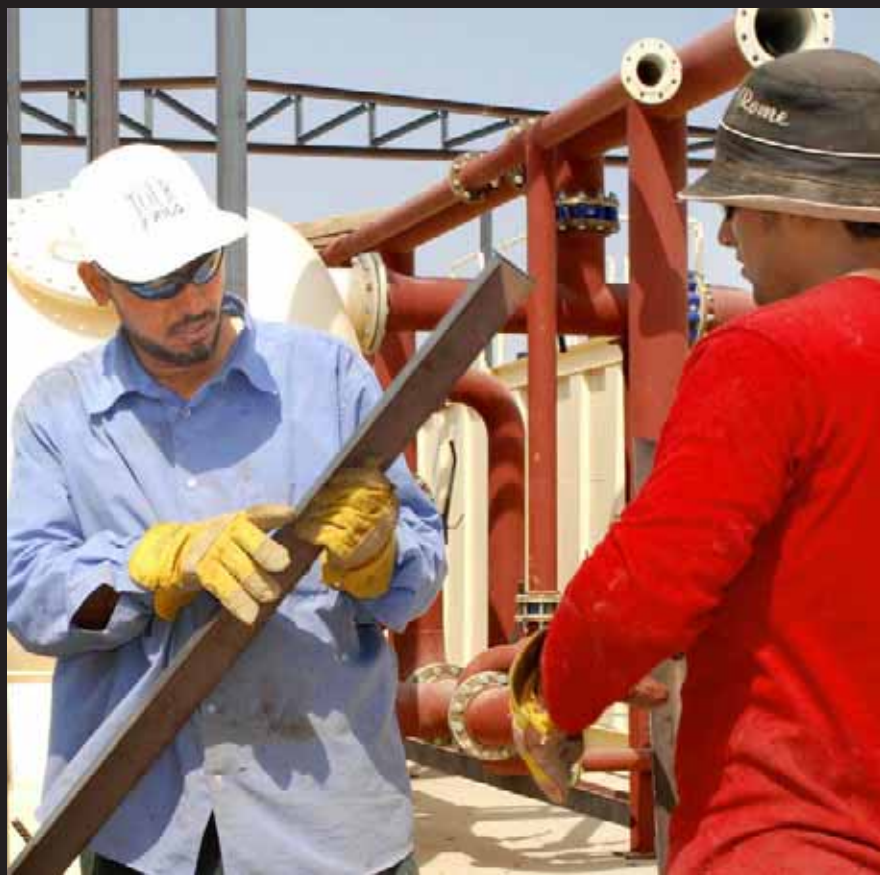
Iraqi crew helps construct additional capacity at Fadiliya's water treatment plant.
