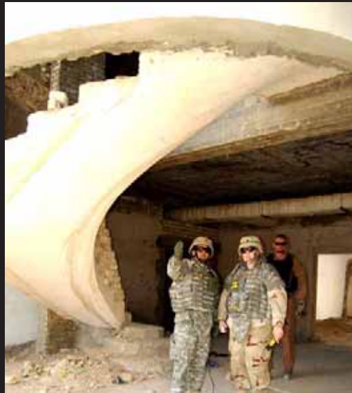
Circular staircase near the main rotunda.
