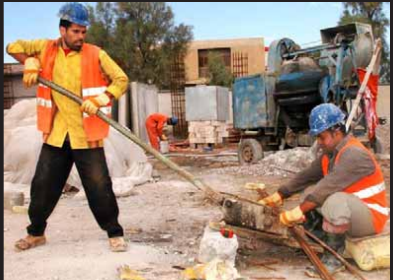
Work continues on a new courthouse project near Basrah.
