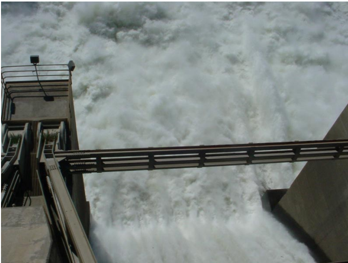
Special spill, 5stops, 8.5k cfs (Bay 5), 45k cfs (total)
