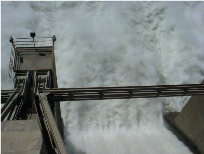
50% spill, 2.5stops, 4.2k cfs (Bay 5), 44k cfs (total)
