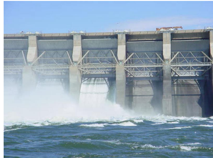
Bulk spill, 8stops, 13.6k cfs (Bay 5), 23k cfs (total)
