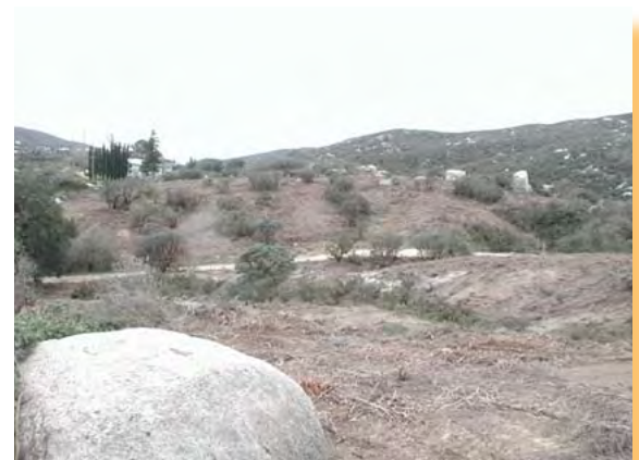
Poppet Flats completed fuel break
