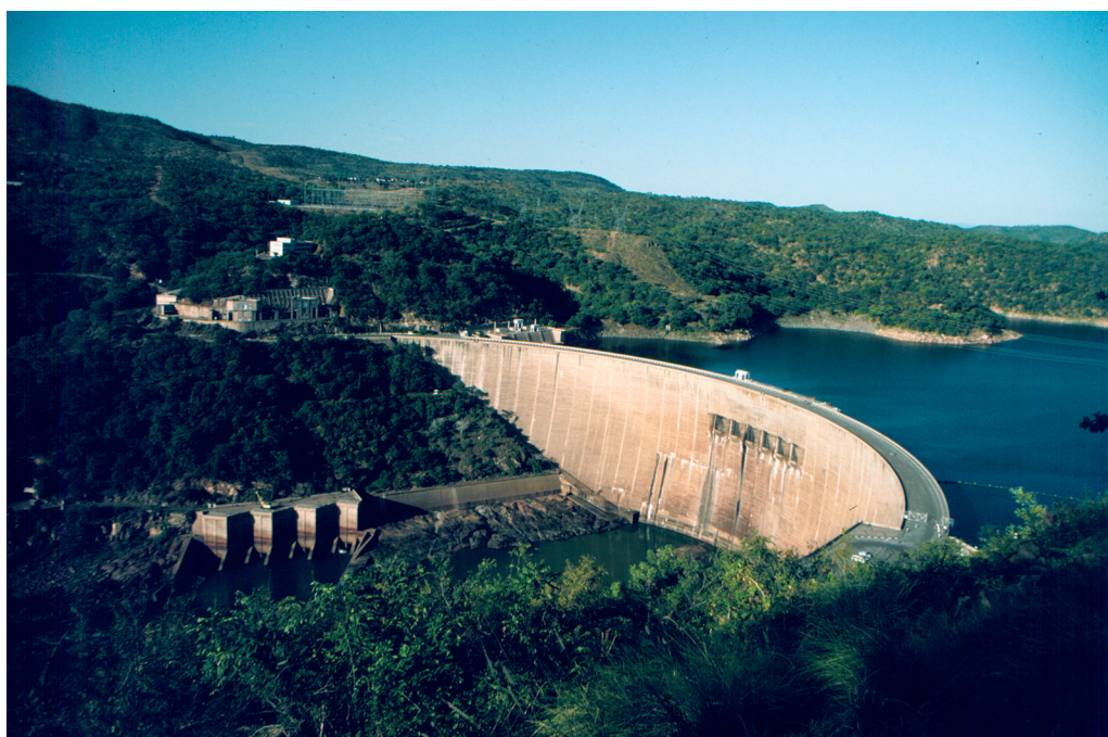
Kariba Dam, Zambezi River. Photo credit: Gordon Matzke.
