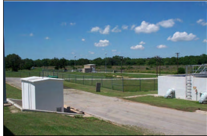
DATE: May 02 DIRECTION: Northeast TAKEN BY: D. Lindsay DESCRIPTION: WWTP located west of wetland site
