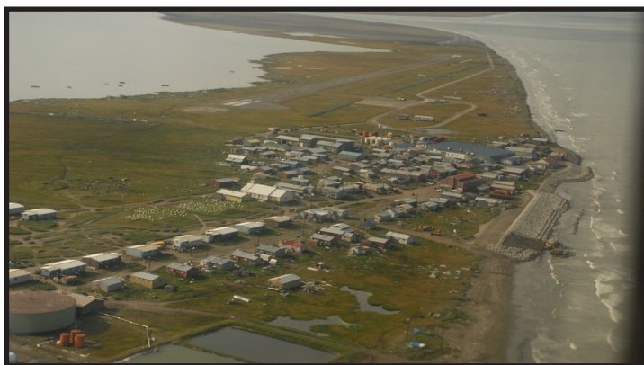
Under a contract with the Alaska District, a contractor places rock revetment at Shishmaref. Coastal erosion threatens buildings, fuel tanks and roads in several remote Alaskan villages.
