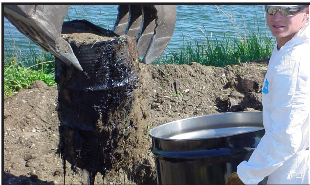
Remediation of drum site at Moses Point
