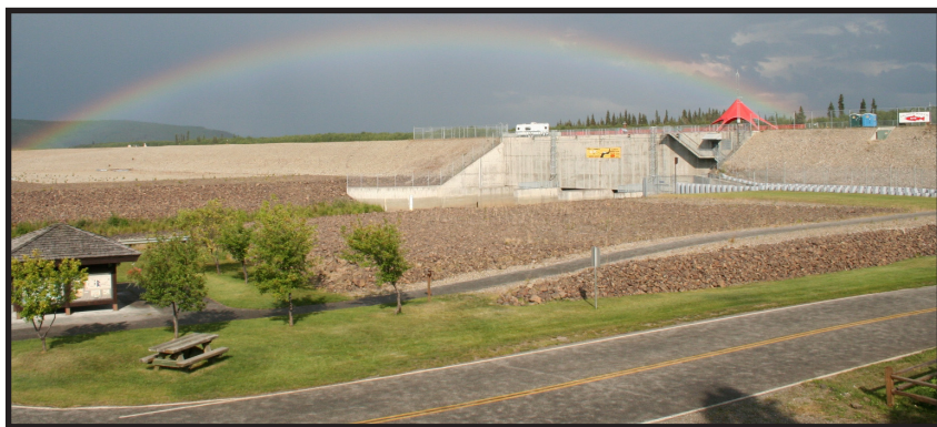
Chena River Lakes Flood Control Project near Fairbanks
