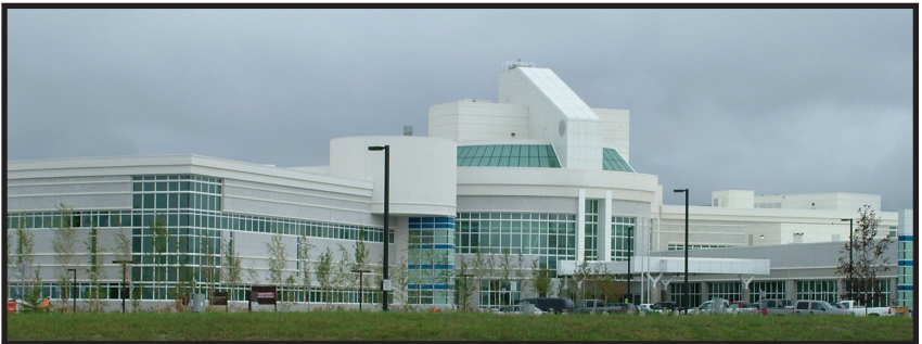
Bassett Replacement Hospital, Fort Wainwright
