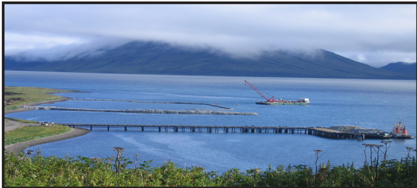
New small boat harbor at False Pass
