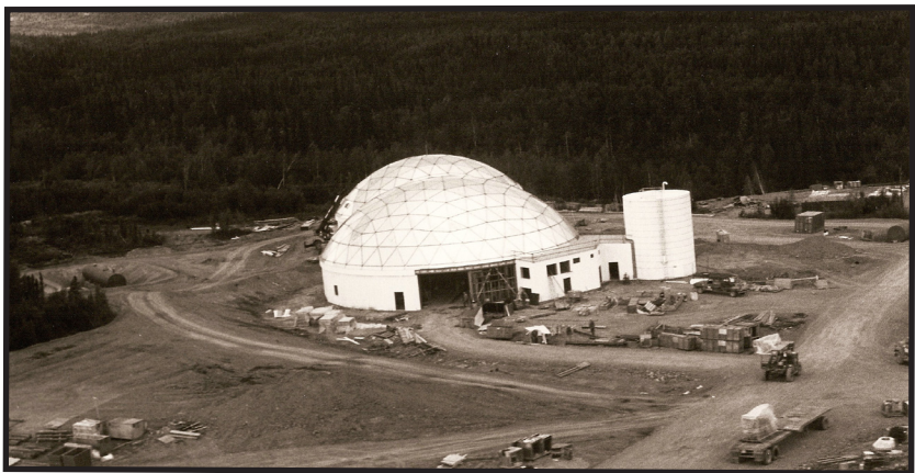
Twin geodesic-domed structures at four Minimally Attended Radar (MAR) sites received a Department of Defense engineering and industrial design award in 1986. The project designed permanent, self-contained shelters for a new generation of radar equipment and living space for personnel.
