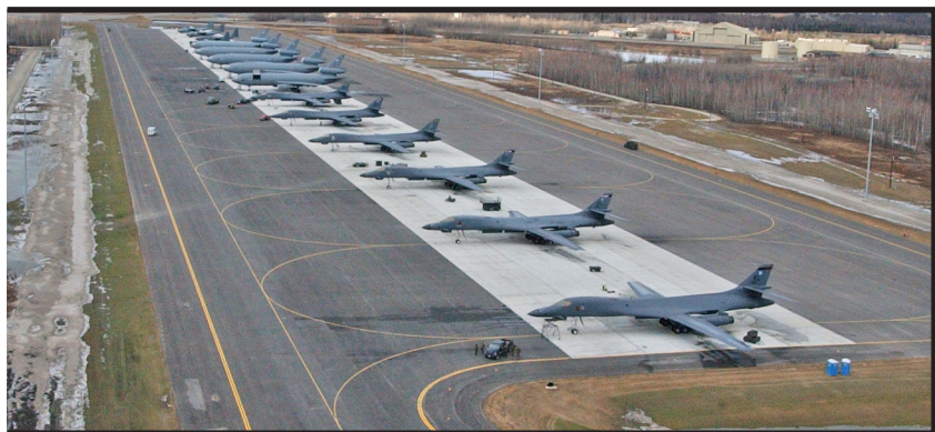
Hydrant fueling system, Eielson Air Force Base
