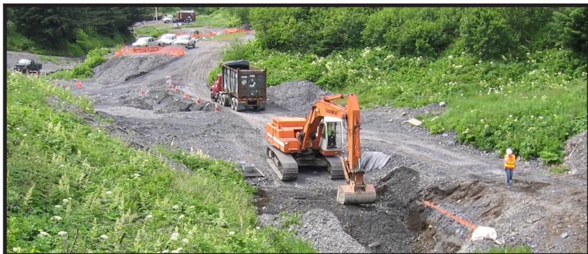
Excavation of PCB contaminated soils in Lower Drury Gulch, Kodiak Island.
